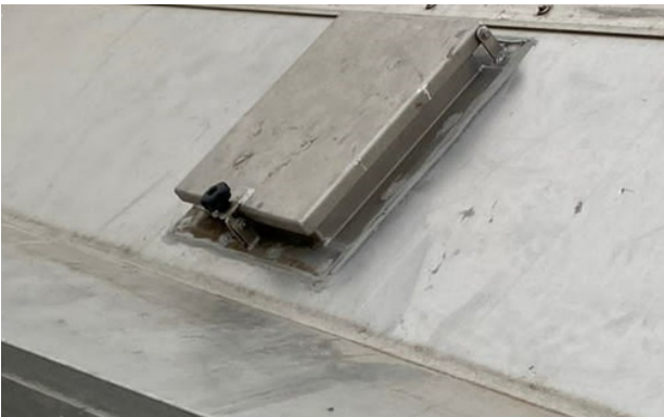
Flashing Inspection Hatch
