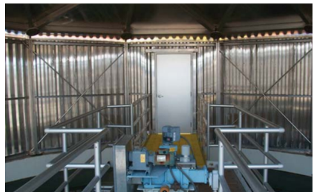
Corrugated Alu Sheeted Side Walls - Inside
