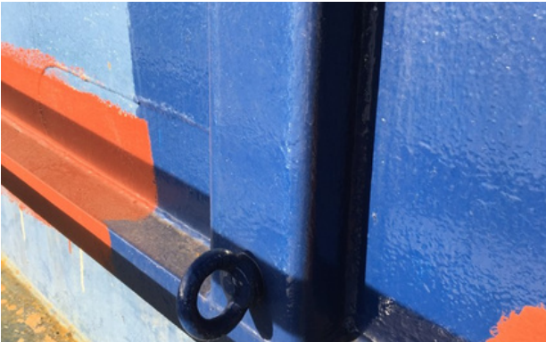
Tank Shell Stiffner
